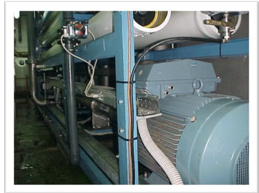
**FEDCO MSS Pump and HPB on Marine SWRO**
